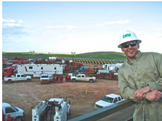
Halliburton preparing a fracking site in North Dakota's Bakken field.
